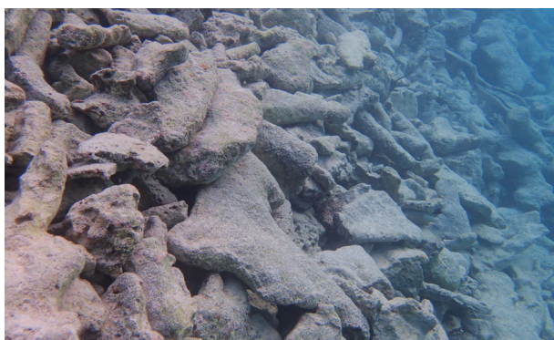
PHOTO 17: REEF RUBBLE JETTY
